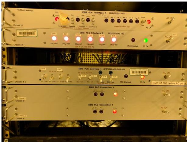
Figure 7: Example of fore pump/ion gauge interface (middle) and PLC distribution (top and bottom). The PLC distribution has rear terminal block connections.
